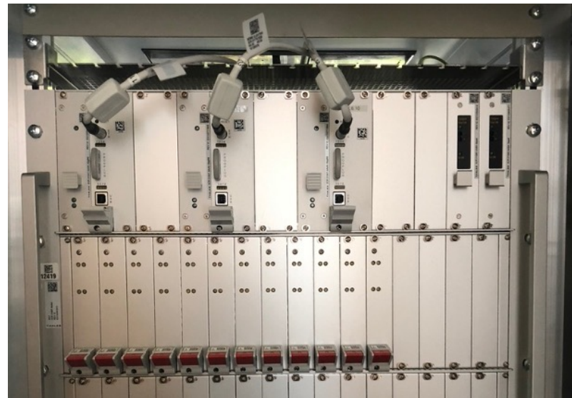
Thales AzLM Axle Counting Object Controller
