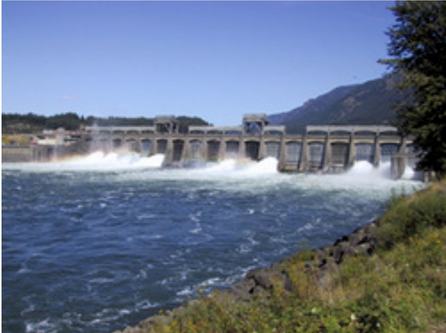
Bonneville Power Authority Dam
