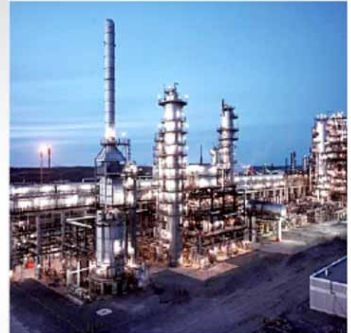
Typical industrial process control plant
